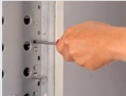
Removing the device bay cover clips
